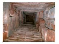
The existing clay flue tiles are removed from the chimney to make room for the new system.
