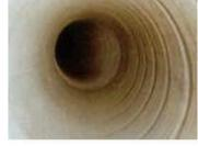
After the mix has set, the former is deflated and pulled out, leaving a smooth, round highly efficient and safe flue passage.
