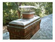
A new chimney cap may be installed to prevent water or animals from entering the system.
