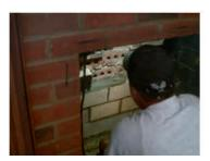
Depending on the condition of the back wall one or all three walls will be rebuilt. (This step varies depending on your
