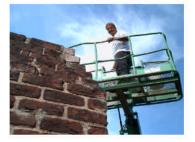
The Supaformer, an inflatable rubber former, is lowered and guided into the clean chimney flue.
