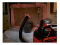
The fireplace opening is sealed off and drop cloths are in place to prevent any debris from entering the room.
