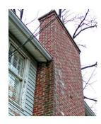
Sometimes if your gutters are full, the overflow of water can spill over onto the chimney and saturate the bricks. Many times there will be evidence of this where the chimney shows signs of stains from the overflow. Therefore, make sure your gutters are clear and not spilling over onto your chimney.
